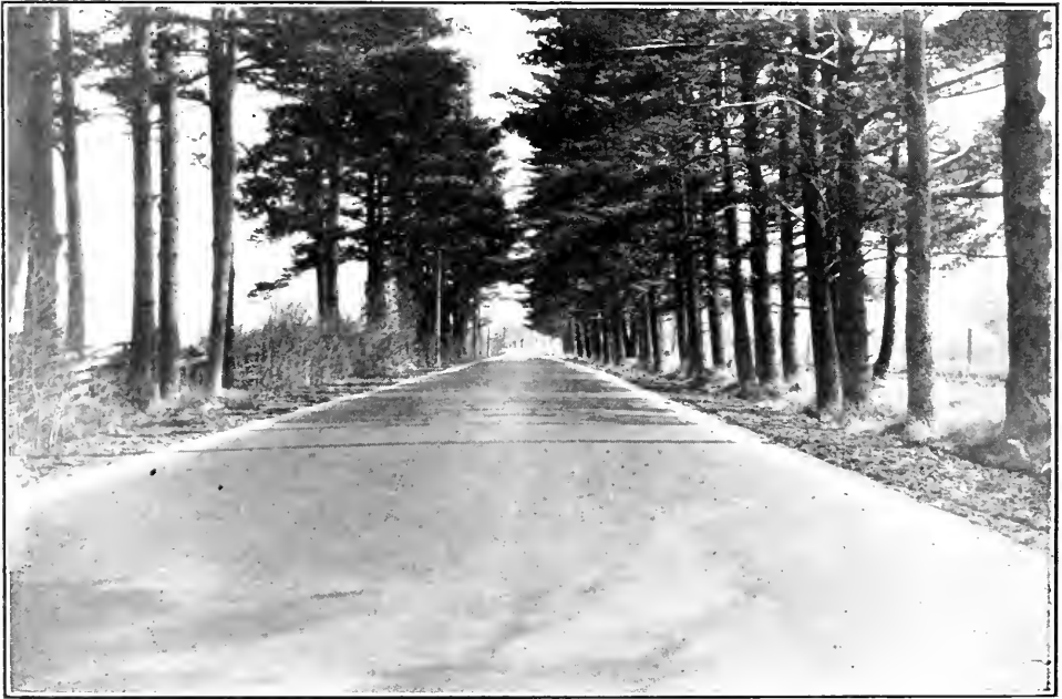
{Black base, sheet asphalt top, Yonge Street, south of Barrie.
